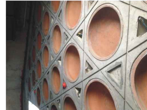
Terracotta pots used as "filler slabs" in Tara building.
